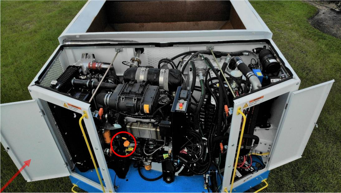
NOTE: The Engine Oil Dipstick can be accessed through the Left Engine Bay Side Door.
